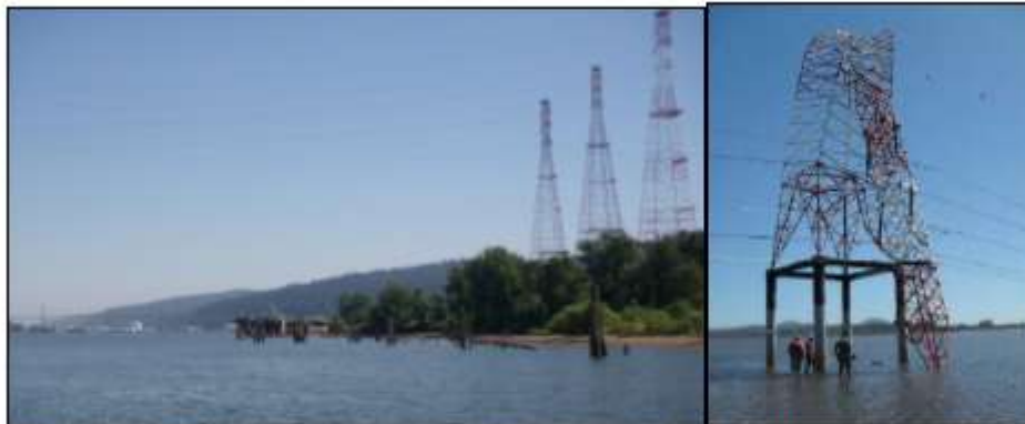
Left: These high voltage electrical transmission towers are built on a river bank in the CEI Hub susceptible to lateral spreading. (DOGAMI photo) Right: Structural damage to a high voltage transmission tower located at a river crossing in 2010 Chile earthquake (Technical Council on Lifeline Earthquake Engineering – TCLEE)
