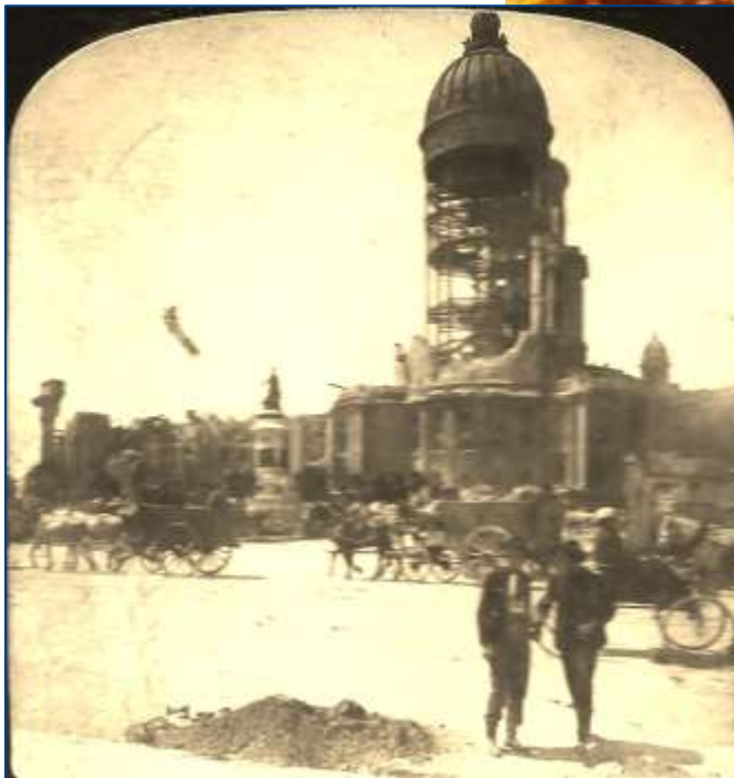
City Hall 1906 Great San Francisco Earthquake
