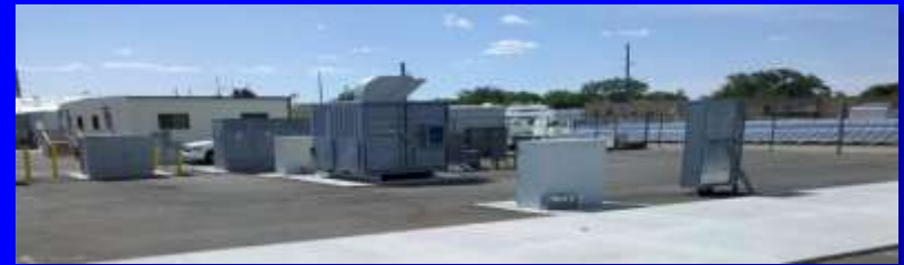
Energy Storage Test Pad (ESTP)
